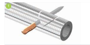
With the longitudinal joint positioned upwards, 2 clean 45° angled cuts shall be made with an initial distance equal to the outer diameter of the Kooltherm® Pipe Insulation section to ensure a proper fit of the branch. When the branch pipe diameter is unequal to the main pipe diameter, refer to the instructions for unequal tees in the next section.
