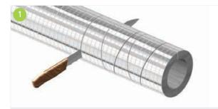
A Kooltherm<sup>®</sup> Pipe Insulation section shall be cut into mitred segments. The width of the mitres shall be determined in order to ensure a good contact with the pipe surface. See the design details of Appendix B for more information. The first and last mitre should have one straight side to match the adjoining straight pipe covers and should have a width of at least 50 mm.
